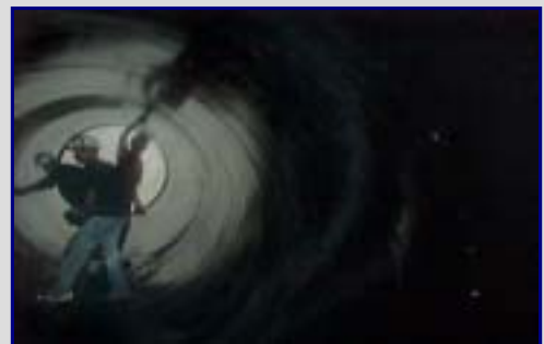
Application of FlueGard™-225S in stack
