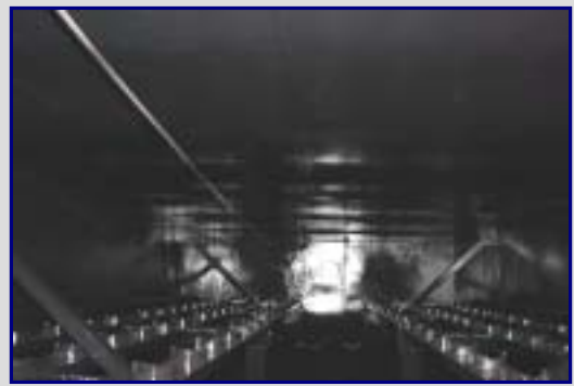
Completed installation of FlueGard™-225S
