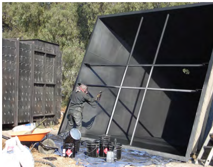
Spray application of CorrosionGard™-160SH2
