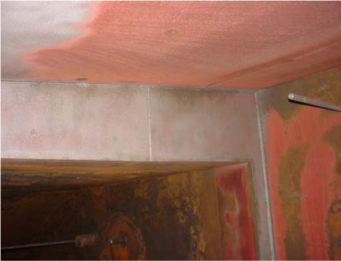
figure 4. Beginning of surface preparation.
