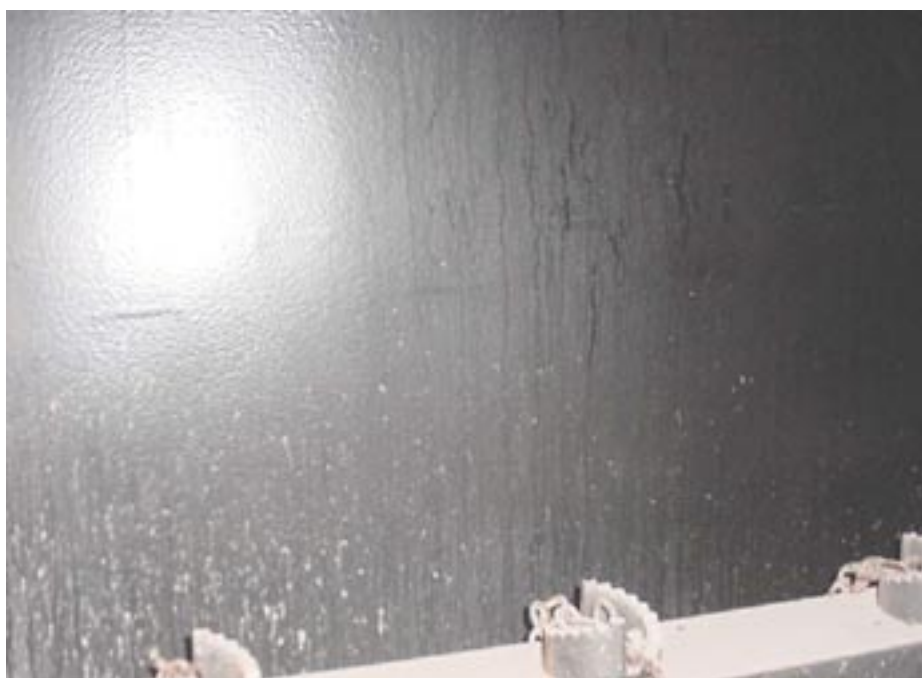
Fig 1. Baghouse wall coated with FlueGard-225SLB, two years previously.
